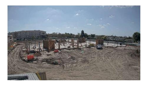
**WESTMONT OF CYPRESS:** The most recent project to break ground is off to a great start! The final mat slab for the main Assisted Living Building will be placed on April 20th while concrete crews are going vertical on Building 1 with shear walls and columns. Slab edge forms have begun on Building 2 with a mat slab pour date scheduled for the first week of May. This project is on schedule to wrap up in the summer of 2021.
