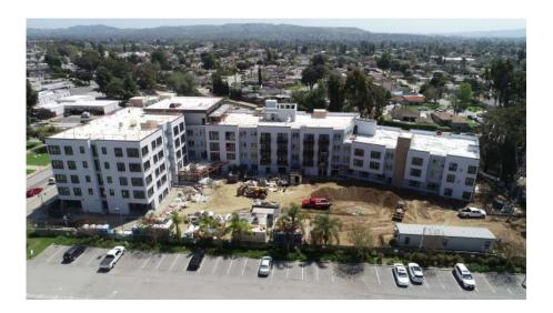
**MERRILL GARDENS AT WEST COVINA:** In West Covina, production drywall is nearly complete and unit finishes are well underway. The exterior is substantially complete with the roof deck landscaping ongoing. Permanent power is scheduled for May 5th which will allow temporary use of the elevators and the dismantling of our OSHA-required man lift. Site work has begun on grade and the project is on schedule for an August completion.
