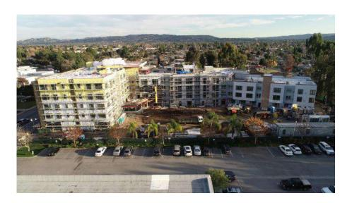
MERRILL GARDENS AT WEST COVINA: At this site, structural framing is now complete, and crews are working to dry-in the roof for drywall and finishes on the east zone of the building. Drywall is well underway in the west and central zones. We are currently scheduled to be complete with roofing activities by the end of January and exterior site work should kick off soon with the underground storm system and grading for the curbs and gutters. This project is on schedule to wrap up in July!
